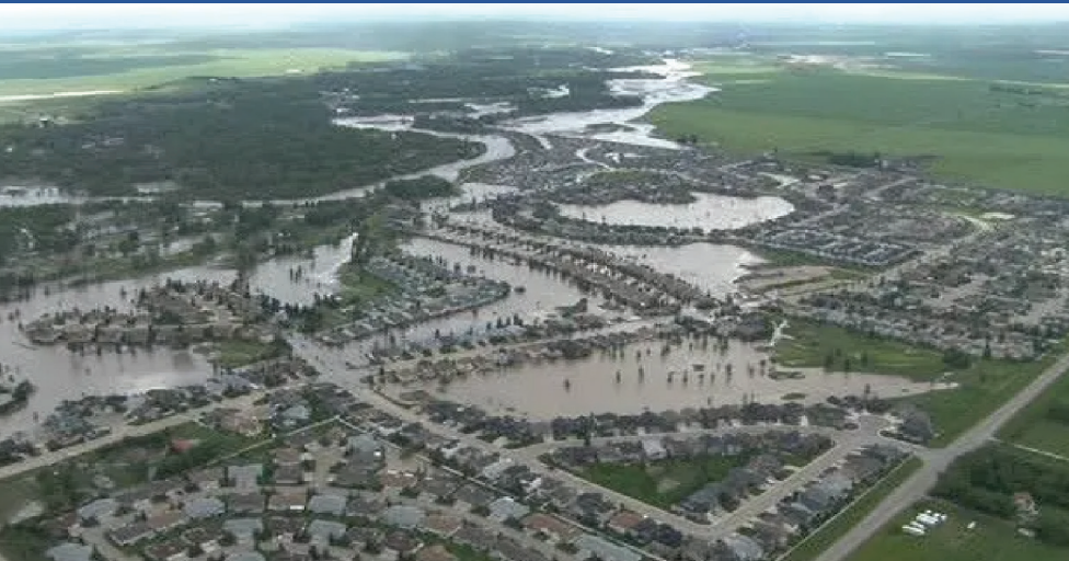
Aftermath of the June 2013 High River flood.
